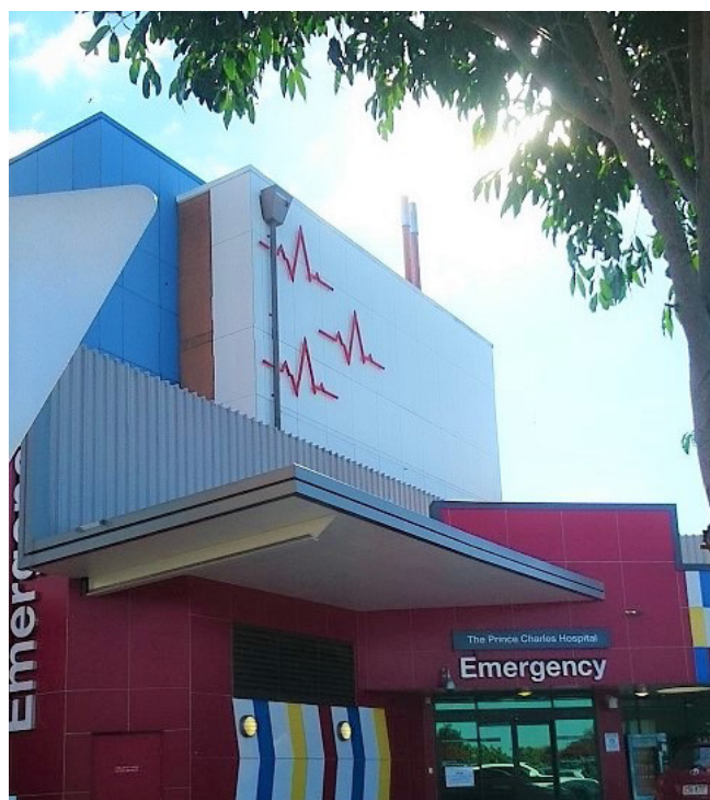
Emergency Department TPCH
