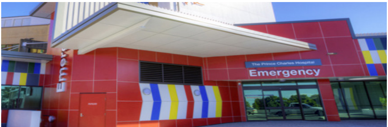
Emergency Department TPCH
