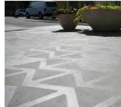
Sandblasted concrete finish paving
