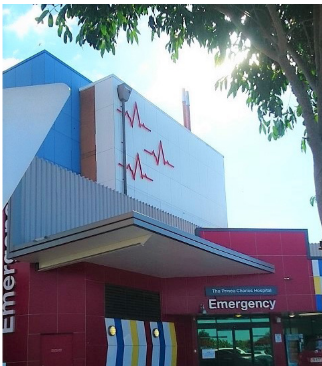
Emergency Department TPCH
