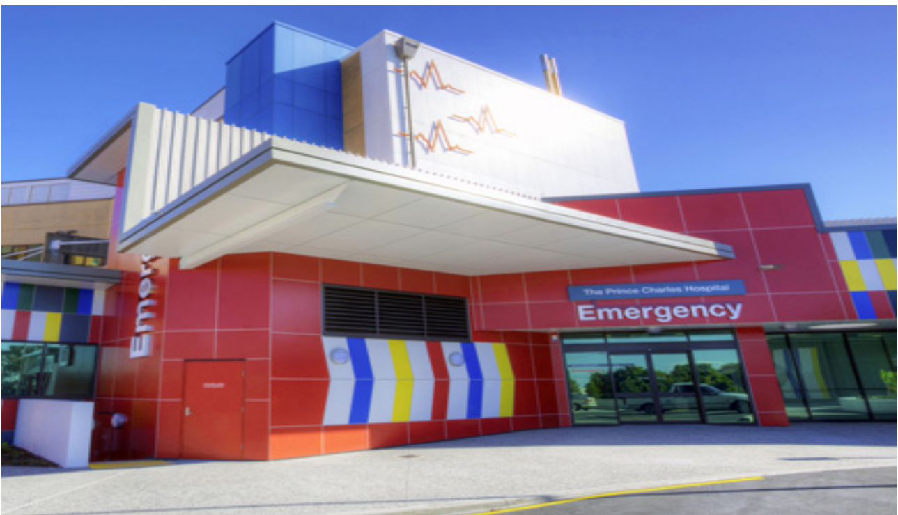
Emergency Department TPCH
