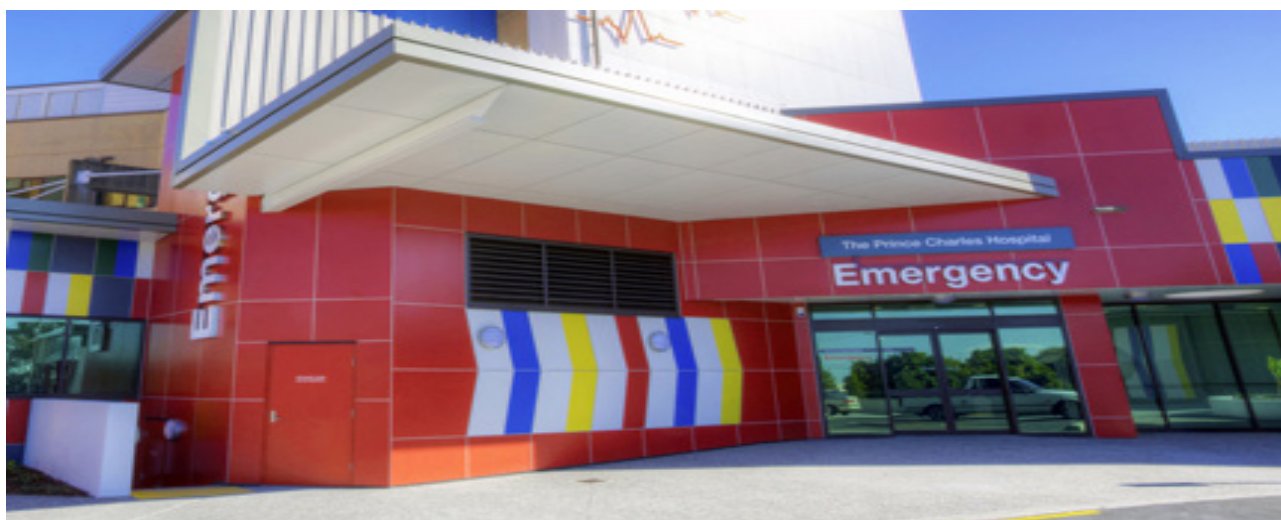
Emergency Department TPCH
