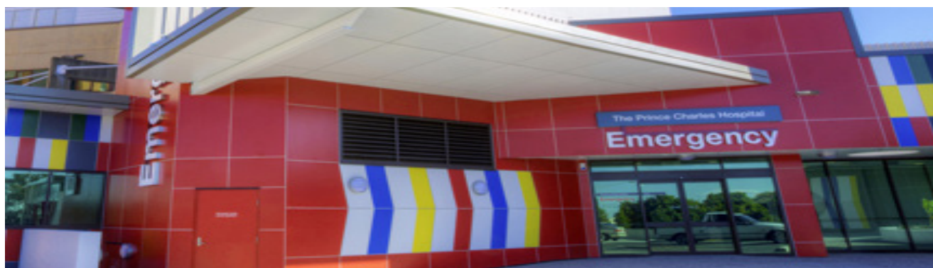
Emergency Department TPCH
