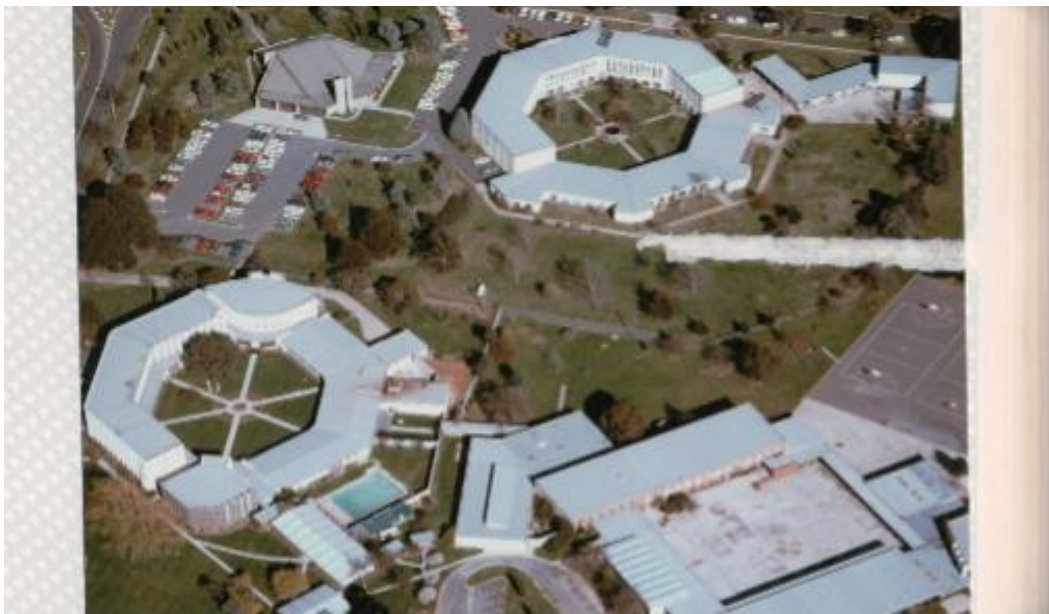
Picture 2: Aerial view of Australian Catholic University, Canberra (Signadou) Campus. Left to Right: Signadou Building, Rosary Demonstration Primary School, Blackfriars Building, and Holy Rosary Parish with spaces for carpark.
